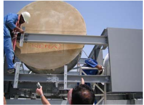
Installation of Screening
