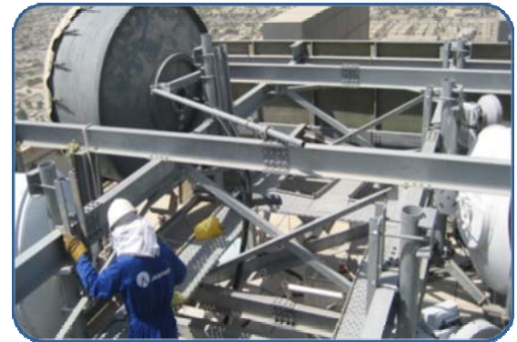
Multiple dishes and antennas installed
