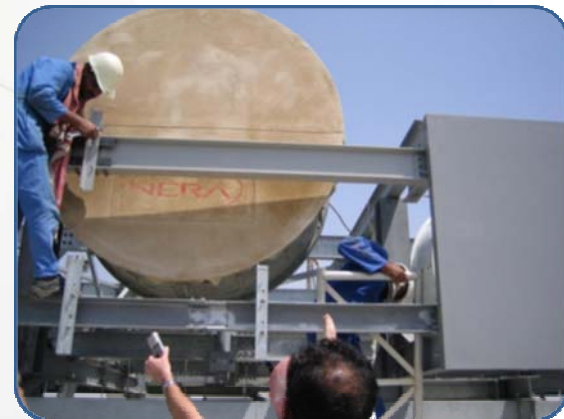
Mounted dish antenna and cladding installation
