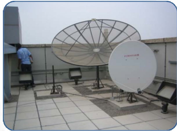
Rooftop prior to installation
