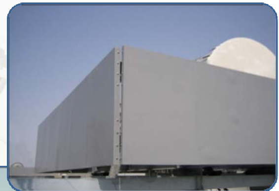
Above: RF Transparent Cladding detail Left: Completed Installation
