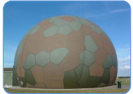
Fig.1 Existing Radome prior to renovation
