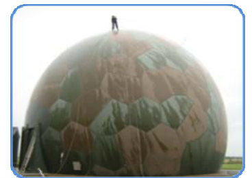
Fig.3 Jet Washing with IRATA trained climbers
