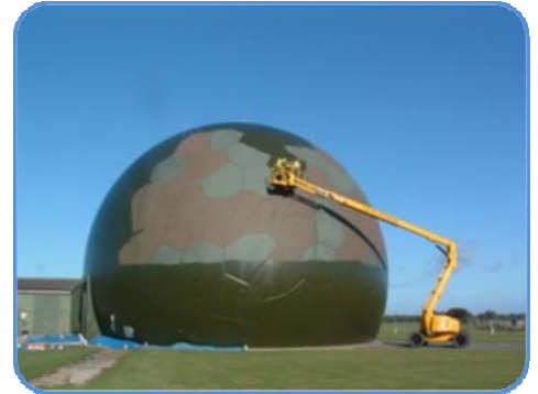
Fig.6 Access Machinery in use
