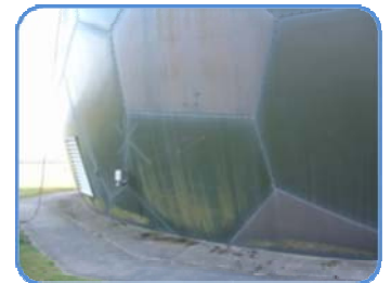
Fig.2 Detail of Radome prior to renovation
