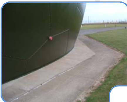
Fig.7 Detail of Radome after renovation
