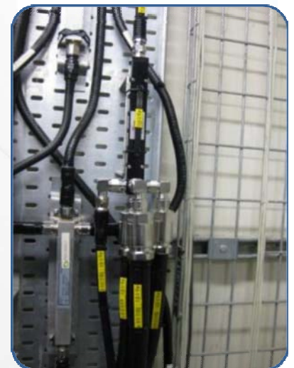
Completed connections and dressed cables
