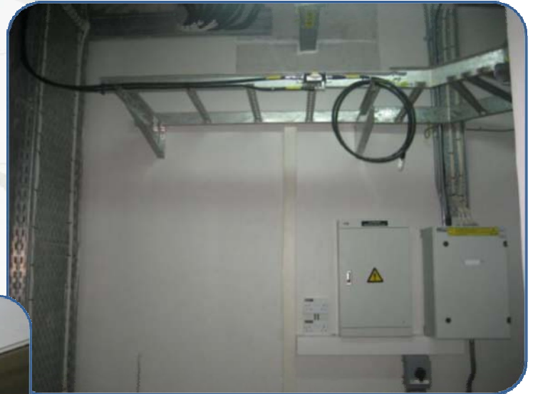
Above: GSM Room electrical fit-out
