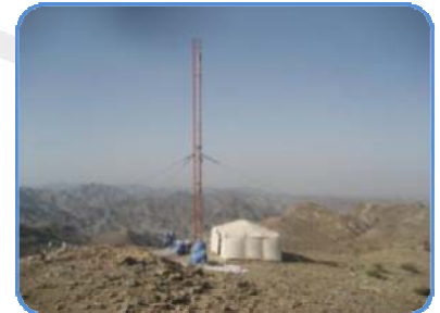
Lower sections and guys installed
