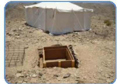
Construction of foundation
