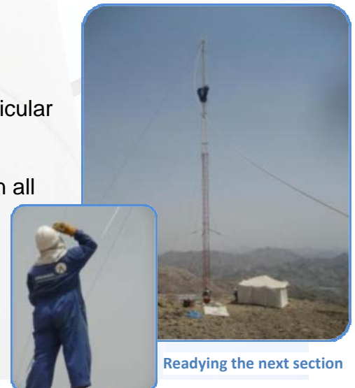
Lower sections and guys installed
