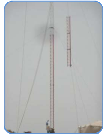
Derrick and Winch in operation
