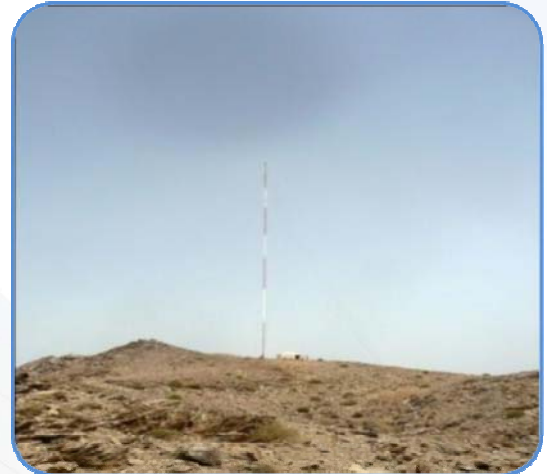
Helimax mast installation - Al Hala
