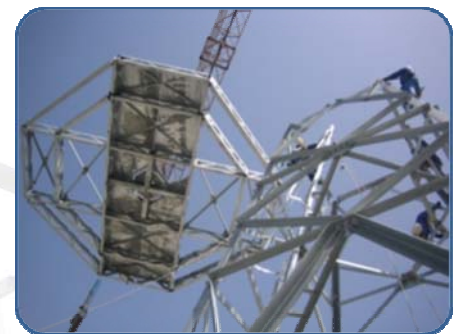
Landing the Tower Platform
