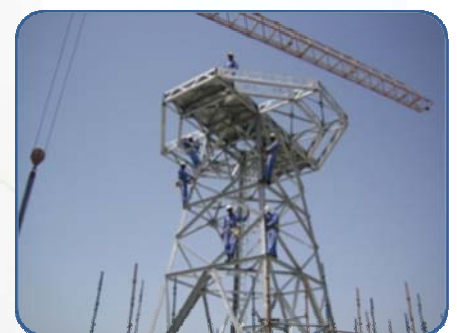
Tower installed on the 160m high rooftop
