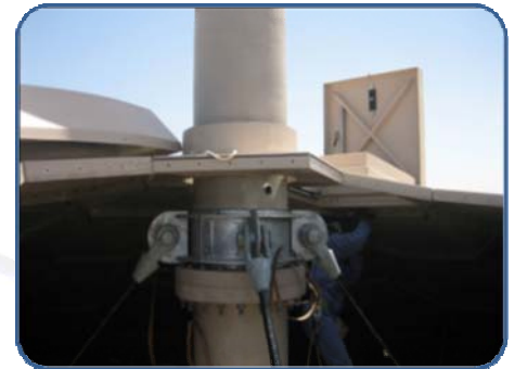
Closing the Radome around the Pinnacle
