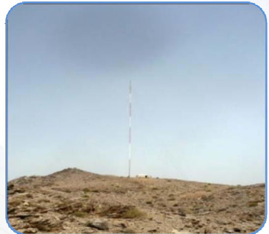
Helimax mast installation - Al Hala
